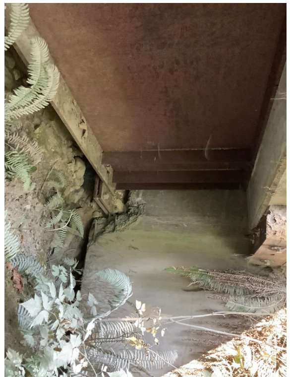
Left Bank Abutment when facing downstream
