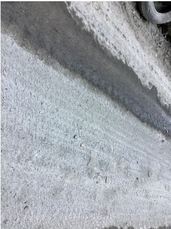
Top of 2nd deck panel
