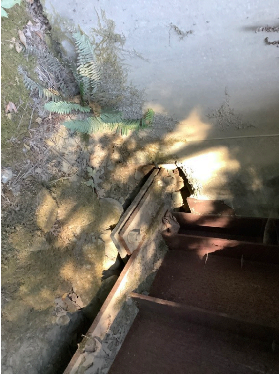
Left Bank Abutment when facing downstream
