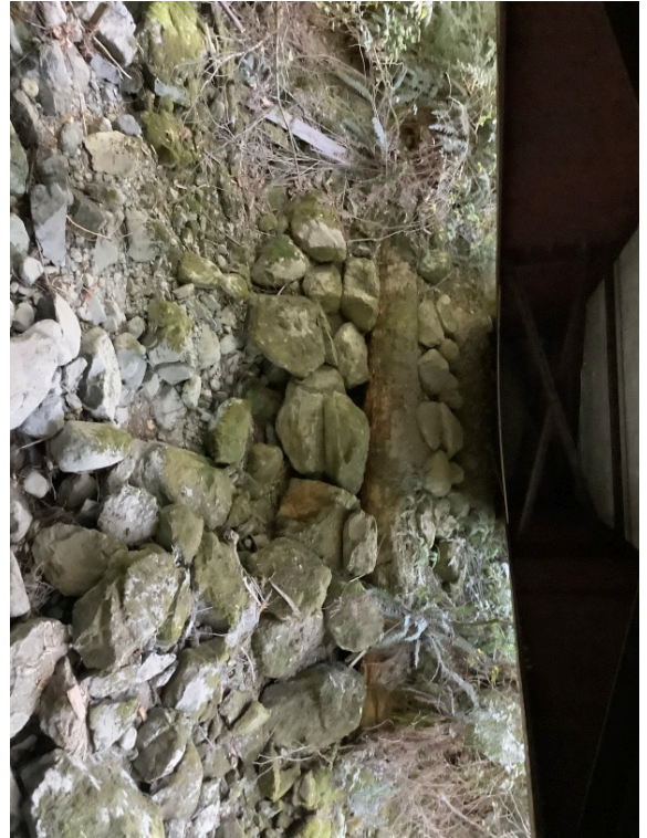
Right Bank Abutment when facing downstream
